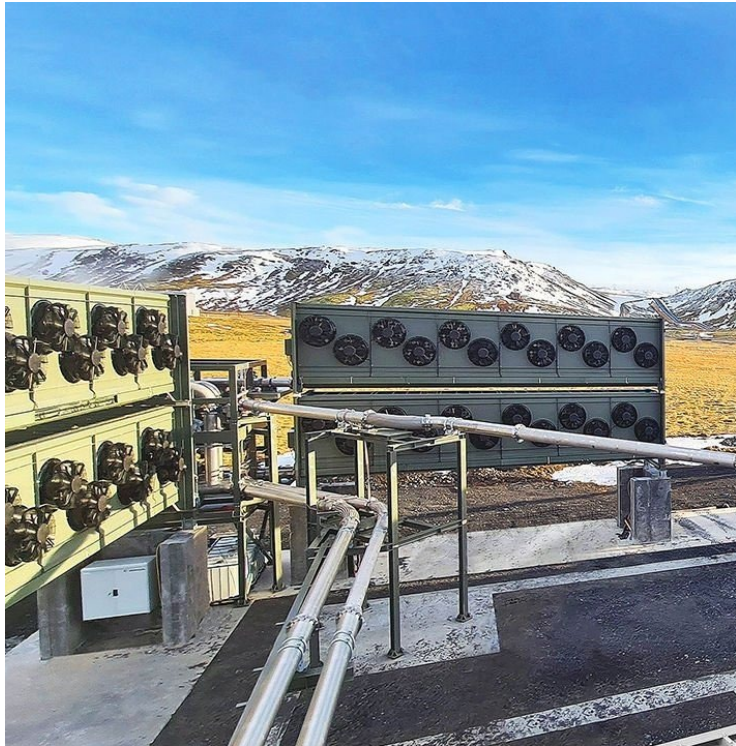
Direct air capture facility ORCA/Climeworks, Iceland Capacity: 4000tCO 2 /year
